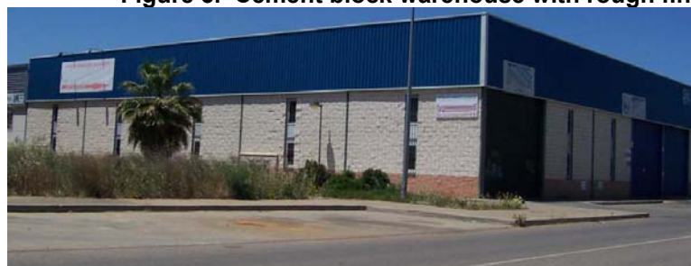
Figure 3. Cement block warehouse with rough finish.
