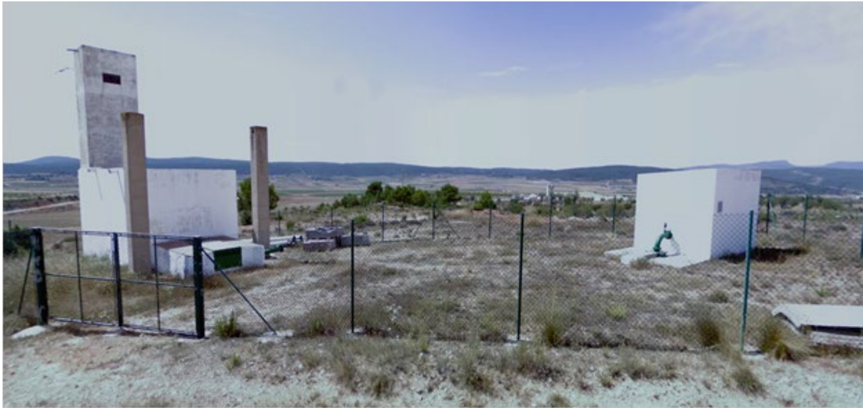
Figure 1. Pumping installation at the starting point of the project.
