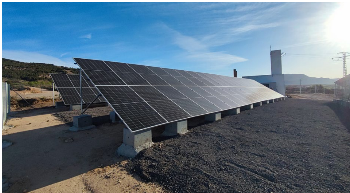
Figure 4. PV installation already finished. Source: own elaboration.
