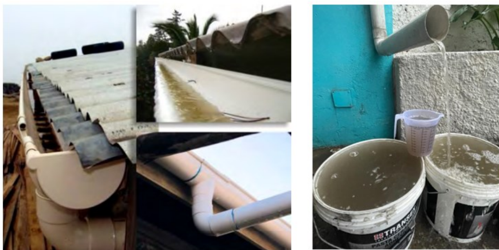
Figure 6: Water collection in experimental work
