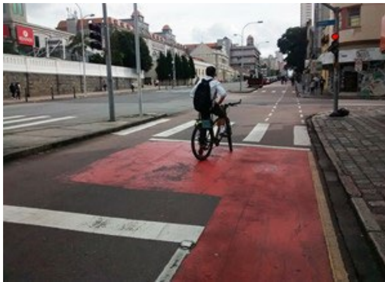
Figure 5: Bicycle lane and bike box installed at the Via Calma - Curitiba.
