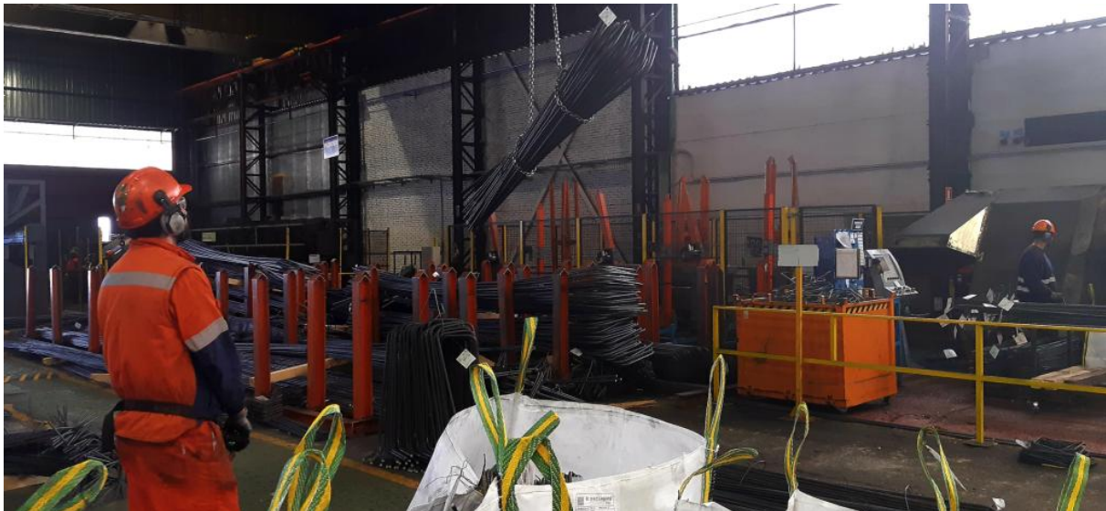
Figure 6: Rebar operations by crane
