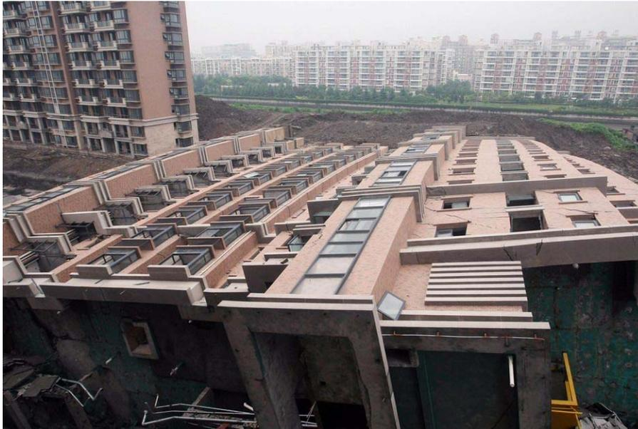
**FIGURA 6 COLAPSO GENERAL DE UN EDIFICIO**
